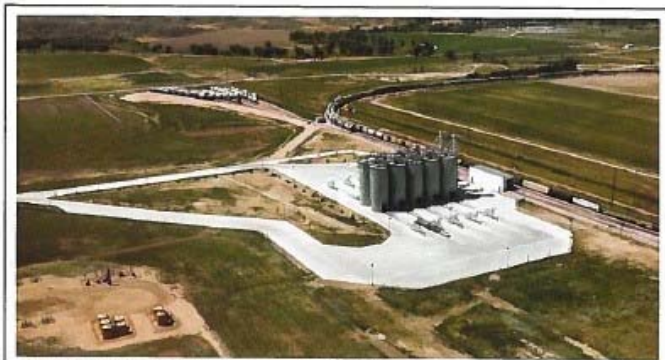
Halliburton delivers 350,000 trucks and 18,000 rail cars of sand each year from facilities such as this sand plant in Windsor, Co., which includes storage for 40 million pounds of sand and has the capability to unload 13 rail cars an hour and load 50 trucks an hour.
